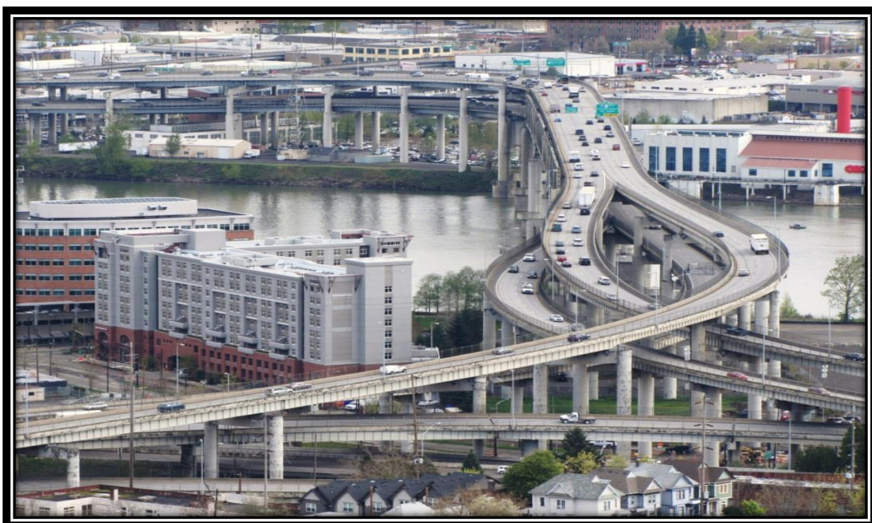
Figure 72: view from Portland Aerial Tram, Portland, OR, USA
