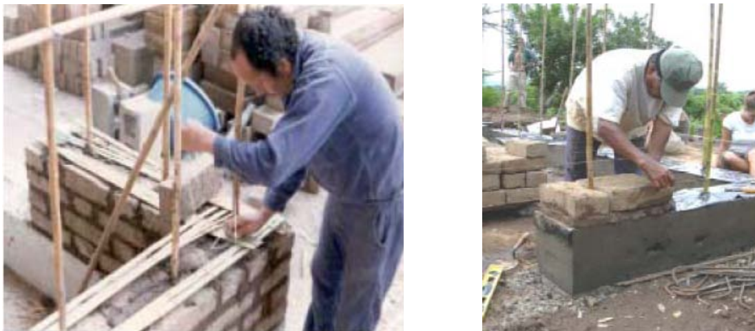
Figure 3-8: Construction with adobe blocks and mortar [81]
