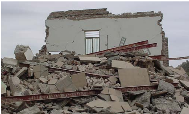
Figure 4-13: Collapse of unfastened slabs [31]
