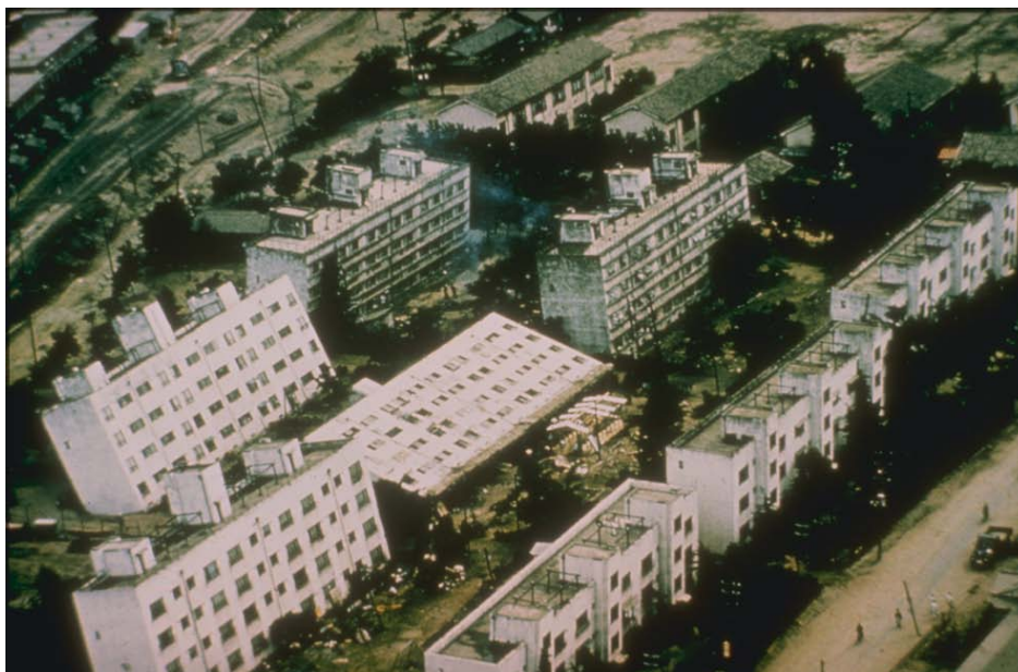
Figure 4-4: Turn over of slim high-rise buildings, Niigata, Japan [16]
