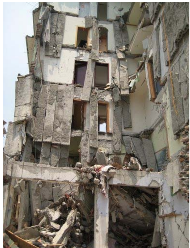
Figure 4-14: Failure of a pre-cast concrete roof in the earthquake in Sichuan, China [34]
