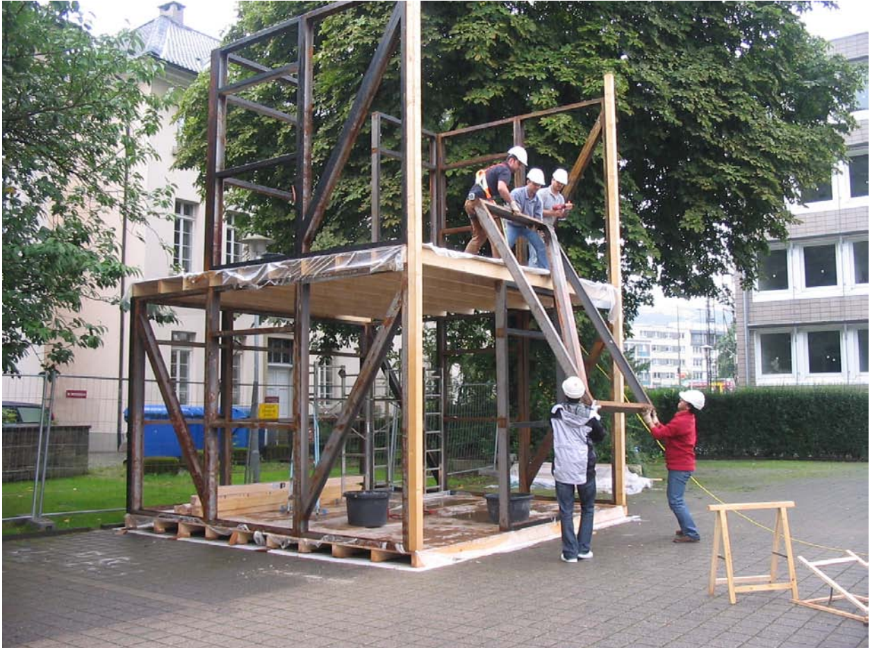
Figure 6-7: Erecting wall panels on site without lifting tool
