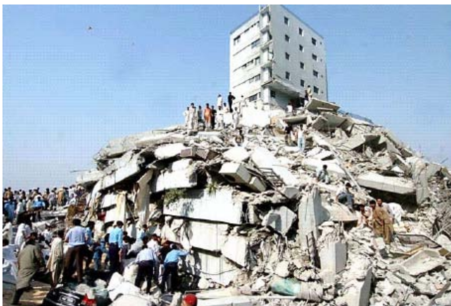
Figure 4-12: Pancake collapse of heavy slabs, Islamabad, Pakistan [AP]
