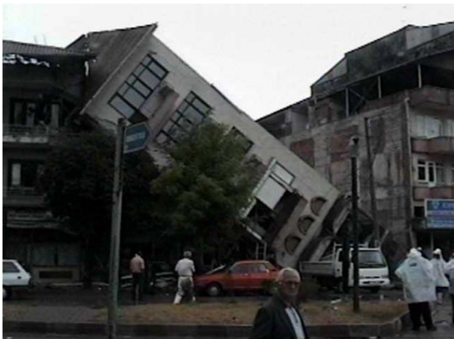
Figure 4-17: Foundation failure of a slim building in earthquake in Adapazari, Turkey [12]
