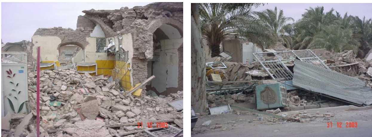
Figure 3-9: Typical adobe buildings destroyed during earthquake in Bam, Iran [Courtesy: Astan-Qods-Razavi]
