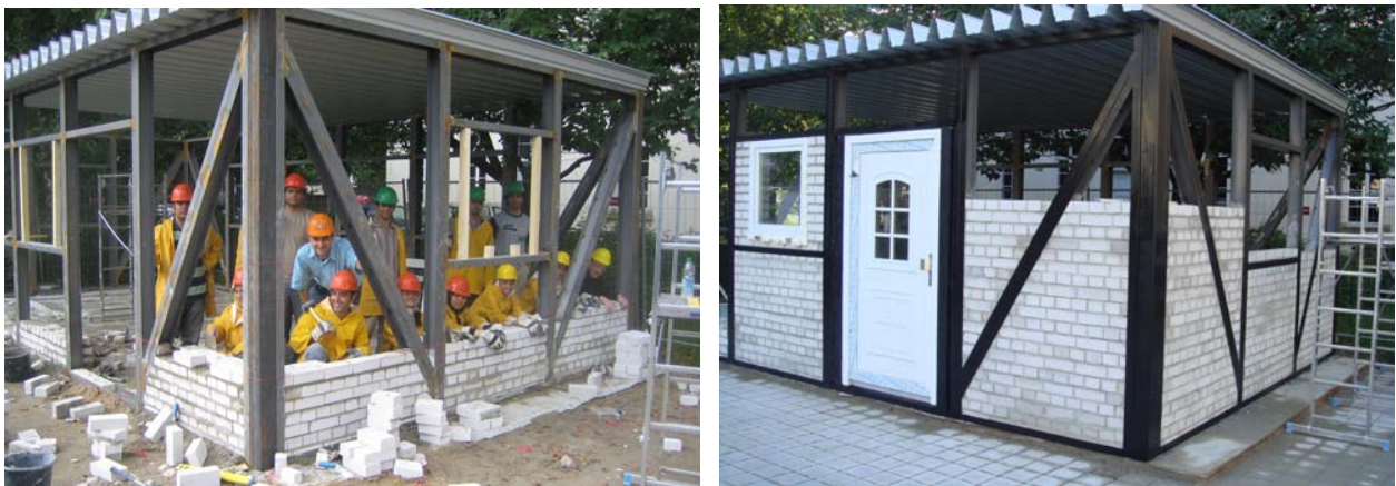
Figure 6-12: Students during work and a view of the final house 2008
