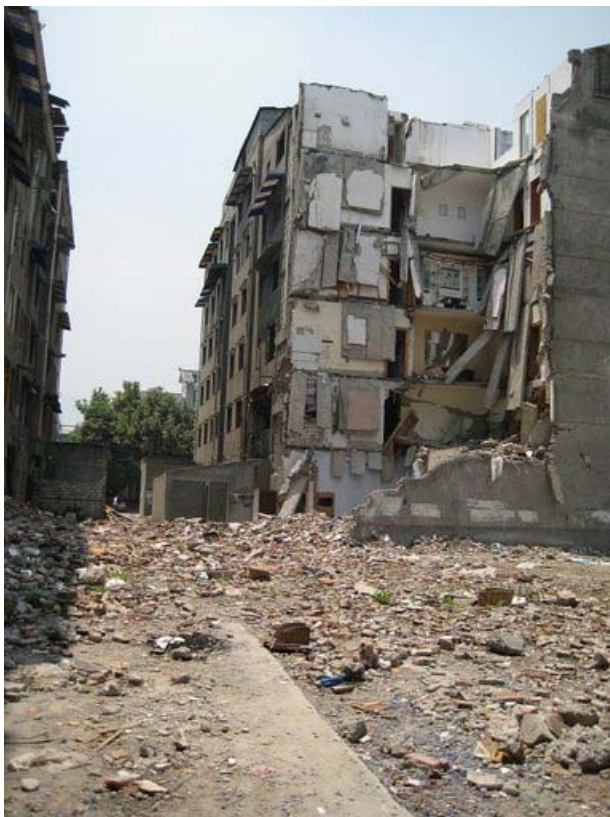
Figure 4-14: Failure of a pre-cast concrete roof in the earthquake in Sichuan, China [34]
