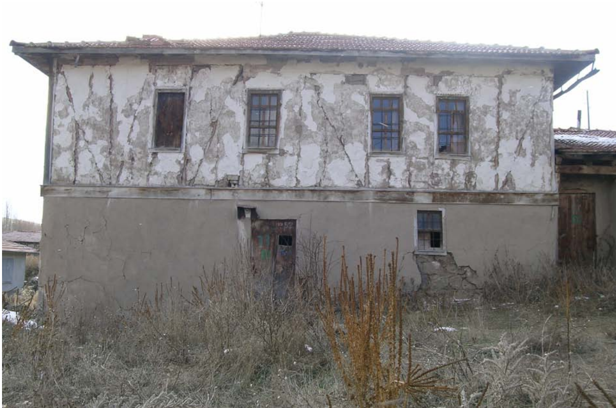
Figure 4-2: A traditional braced house withstood an earthquake of magnitude 5.9 on the Richter Scale in Yuva Village, Cankiri Province, Turkey [14]
