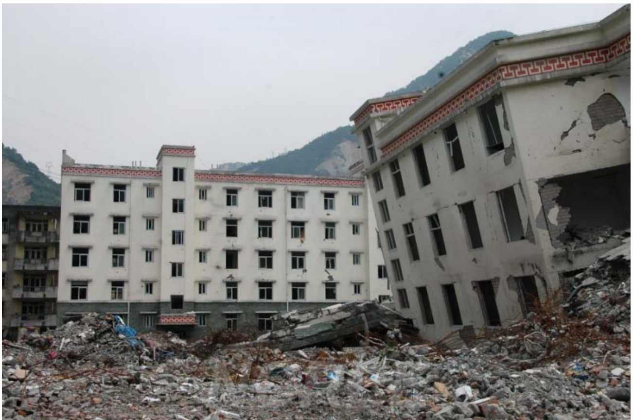
Figure 1-1: Collapse of school buildings in Wenchuan, China during the M 7.9 earthquake of May 12, 2008 [13]
