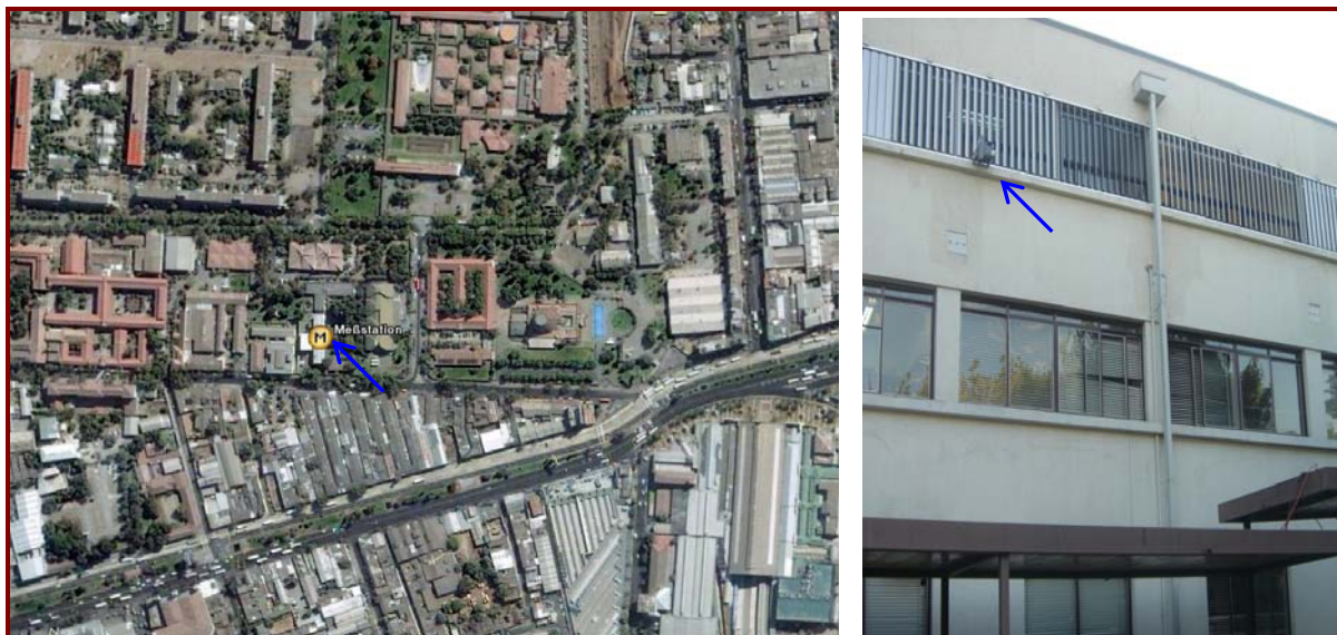
Fig. 6.1.2: USACH Measurements site at the University of Santiago de Chile (left). Measurements took place at the third floor of the physics department building (right).
