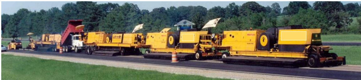
Fig. 15: Hot in-place recycling using remixing process. ( http://martec.ca/benefit/ . Last accessed 26.09.2018).
