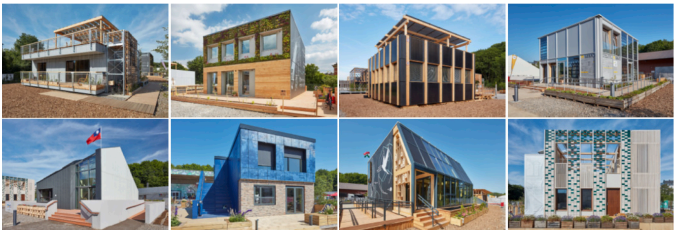
Fig. 1. The Wuppertal cluster buildings simulated in this work (Ref: © Sigurd Steinprinz, University Wuppertal).
