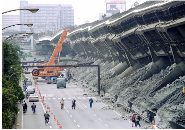
Figure 1.1: Pier failure of a road bridge, Earthquake Kobe 1995 1
