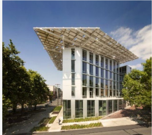
(6) Bullitt Center. Source: [126] Photo Credit: International Living Future Institute
