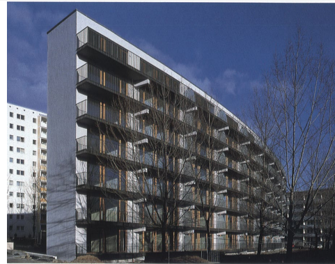
(1) Low Energy Apartment Building. Source: [118] - Photo Credit: Christian Gahl, ASS-Archiv
