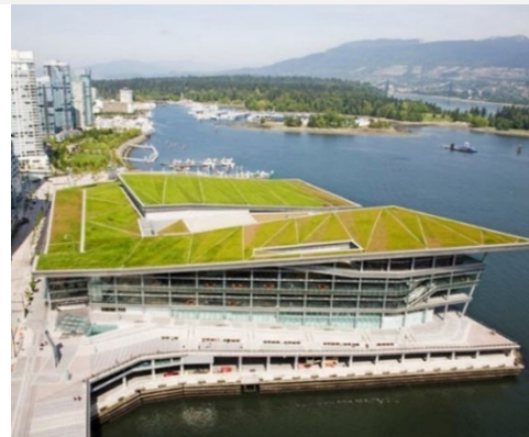
(3) Vancouver Convention Centre. Source: [124] Photo Credit: Nic Lehoux
