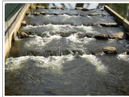
(B) Aeration on a cross-bar block ramp due to local hydraulic jumps OERTEL AND BUNG (2012A)
