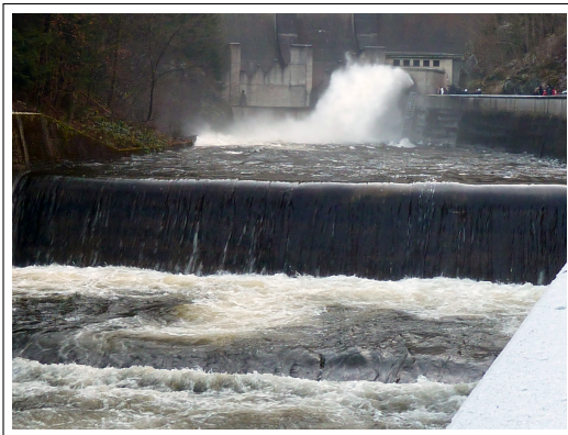
(A) Aeration at a weir downstream of Oker dam in Germany; note the strong aeration at the bottom outlet in the background
