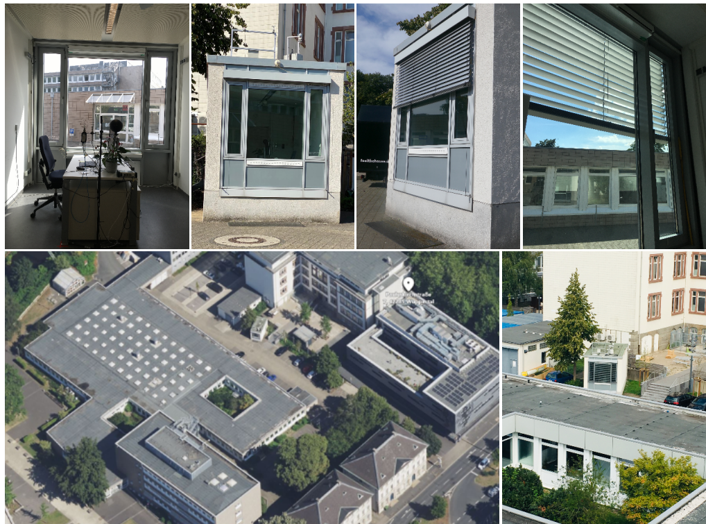
Figure 4.1: "btga-box" test facility aerial, exterior and interior views.
