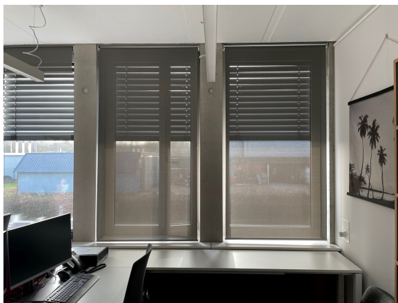
(a) Interior view of the "double shading"
